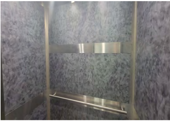
25 Elevator Cab Walls
