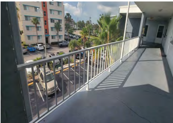
37 Walkway Railing Overview
