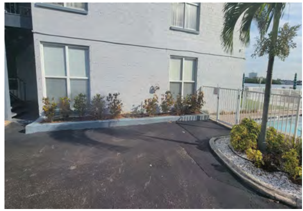
2 Right Side of Building
