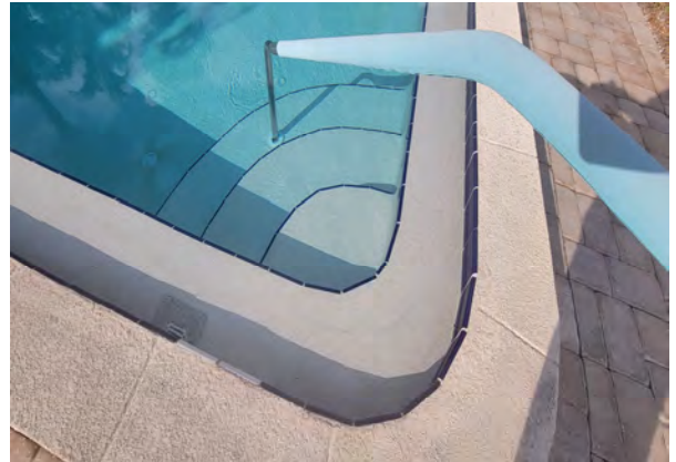
12 Pool Stairs and Handrail
