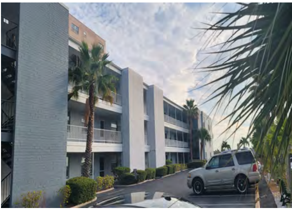
1 Front of Building
